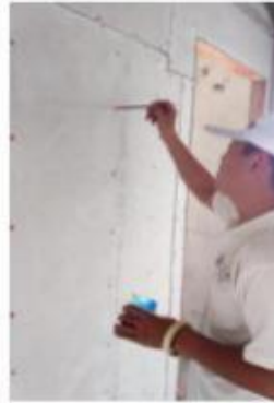
Anti-corrosive treatment
