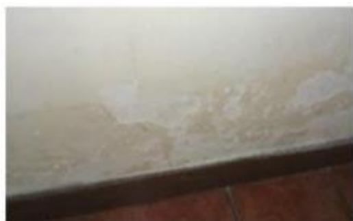
Powdered old wall surface
