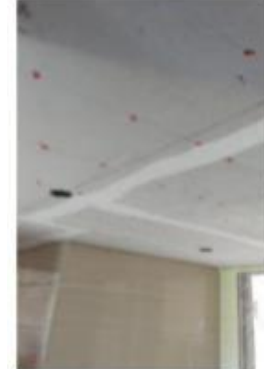
Joint patching treatment
