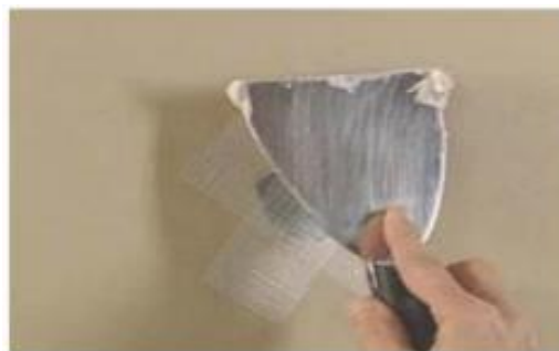
Crack-proof mesh to fill holes
