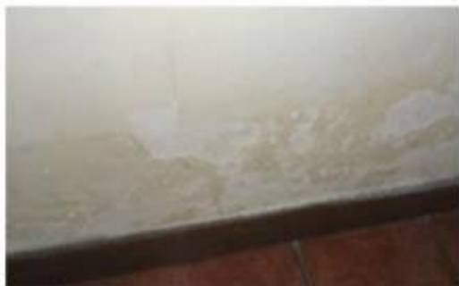
Powdered old wall surface
